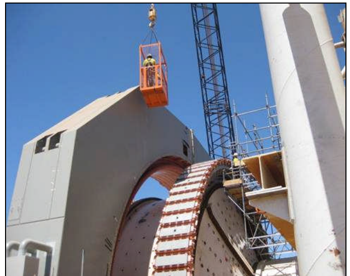
Figure 1. Gearless Mill Drive.
