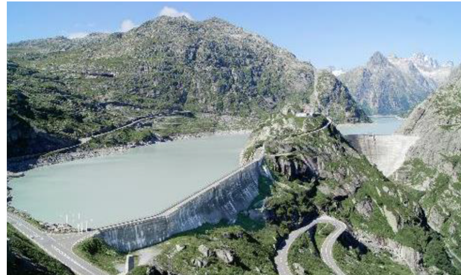
Image: ABB (Grimsel II, Switzerland) Pumped Hydro Energy Storage 26 February 2019.
